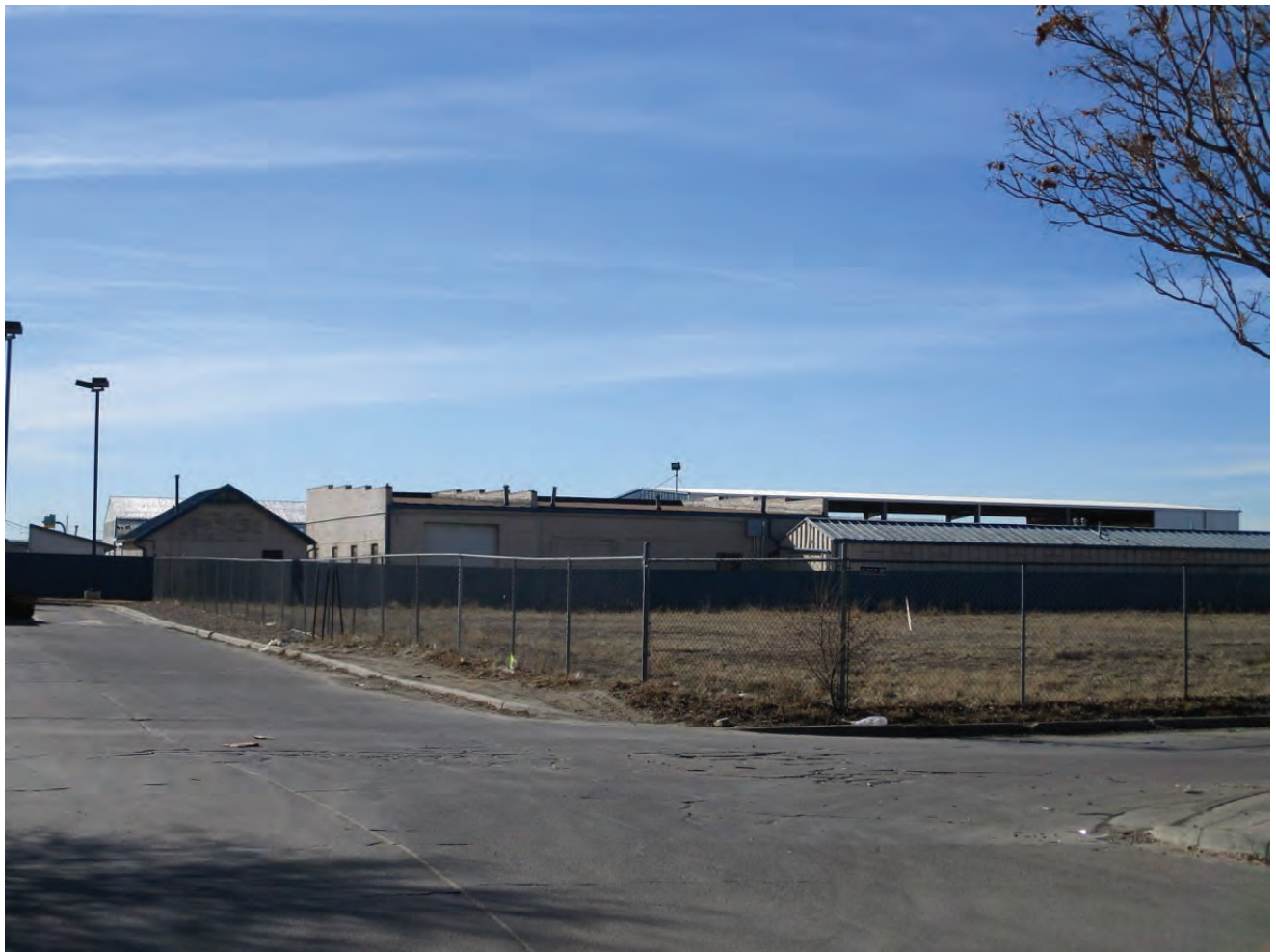
5AM4071_3.jpg: Looking south at 5AM.4071 from driveway on north adjacent site (January 24, 2020)
