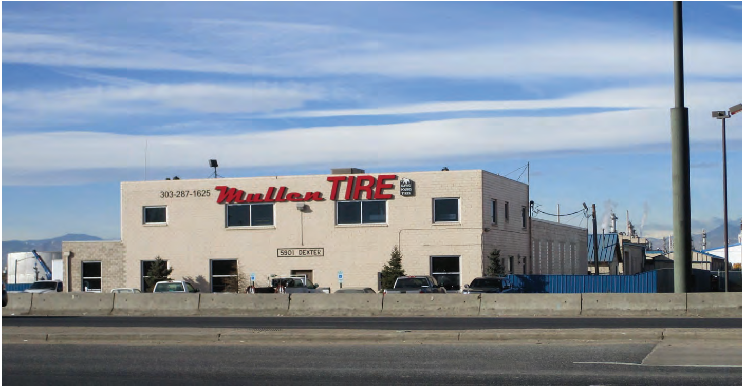
5AM4071_1.jpg: Looking west at 5AM.4071 from Vasquez Blvd. (January 24, 2020)
