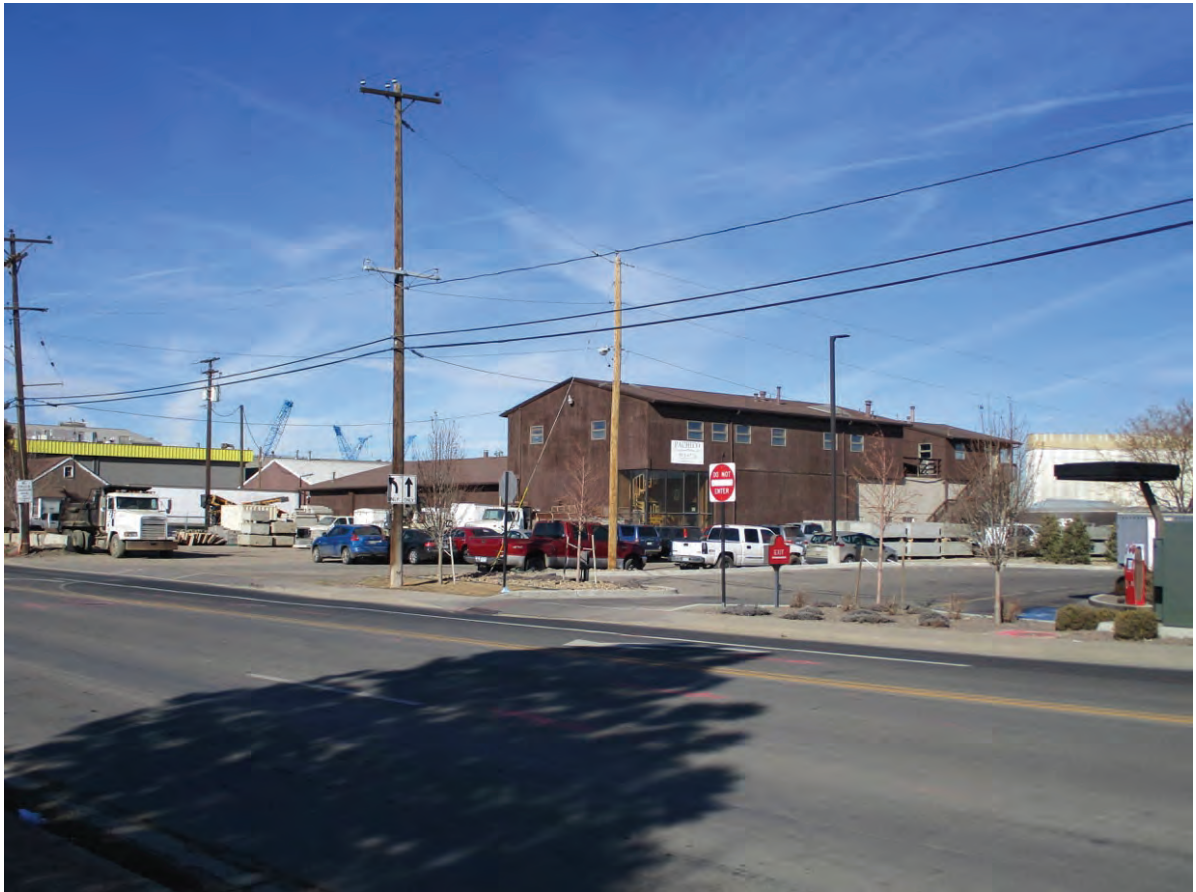
5AM4074_3.jpg: Looking northwest at 5AM.4074 from E. 60 th Ave. (January 24, 2020)
