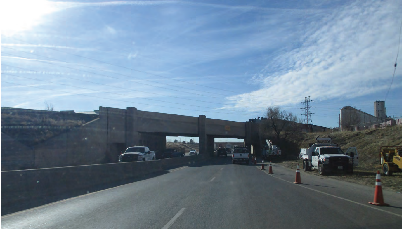
5AM3924.3_3: Looking south along US 6 north of railroad overpass (January 24, 2020)
