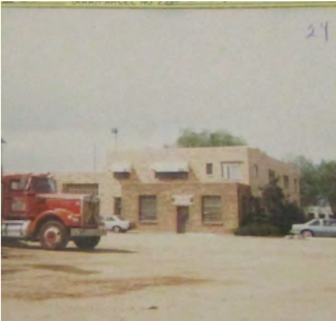
Image of property from Adams County Assessor (date unknown), looking west at main building
