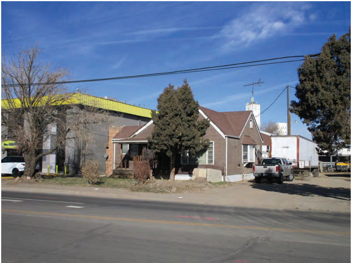
5AM4074_2.jpg: Looking northwest at 5AM.4074 from E. 60 th Ave. (January 24, 2020)
