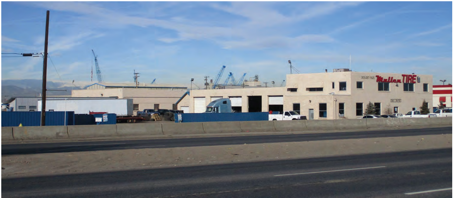
5AM4071_2.jpg: Looking northwest at 5AM.4071 from Vasquez Blvd. (January 24, 2020)
