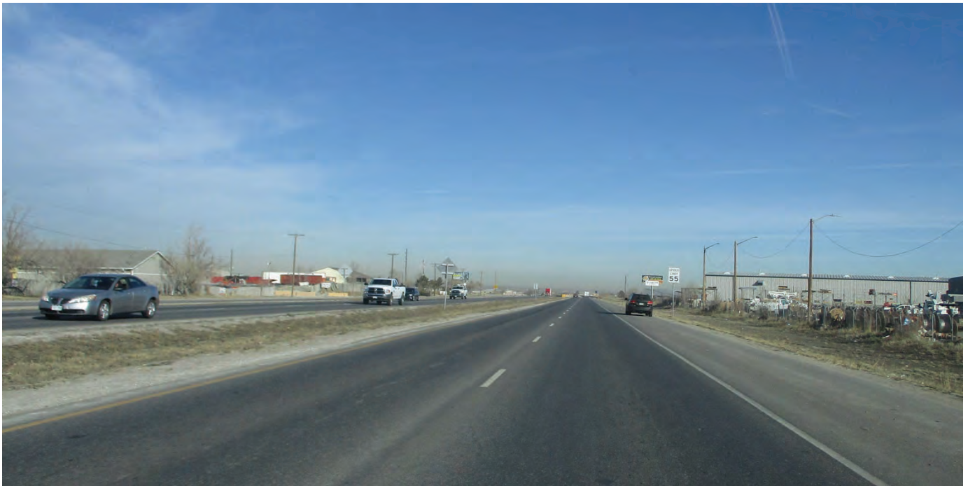
5AM3924.3_4: Looking north along US 6 north of the intersection with 77th Ave.
